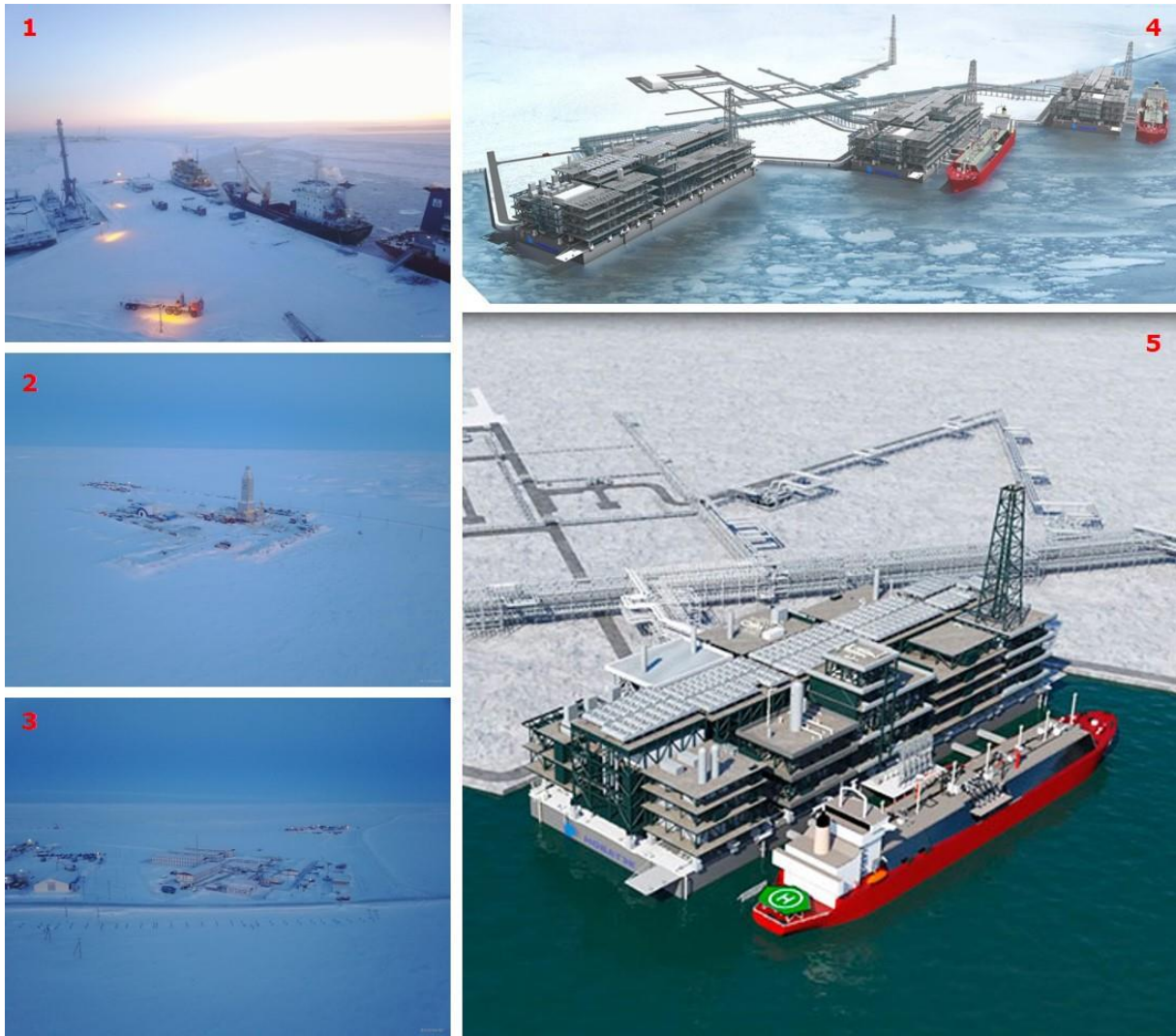
Figure 6: General view of the main Project facilities:
